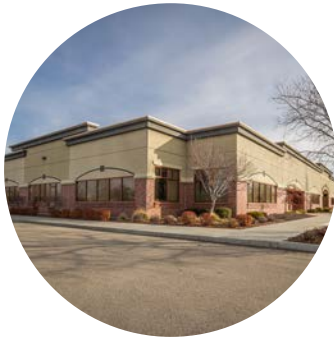
SIERRA PLAZA 9,537 SF | OFFICE FOR LEASE | TENANT REP
