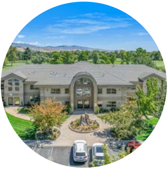
RIVERSIDE BUSINESS CENTER 7655-7669 W, RIVERSIDE DRIVE, BOISE, ID 83714 LANDLORD REPRESENTATION
